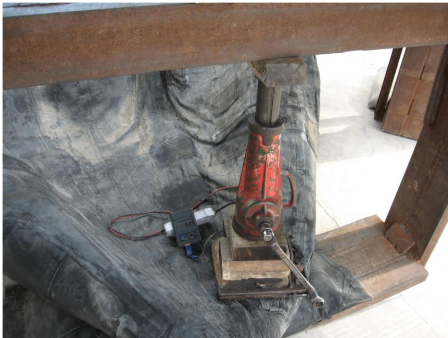
Fig 1.5 Heating up temperature 135°C; waiting period 40 ~ 50 minutes
